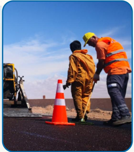
As shown side, the slurry seal maintenance extends the life of the coating significantly.
