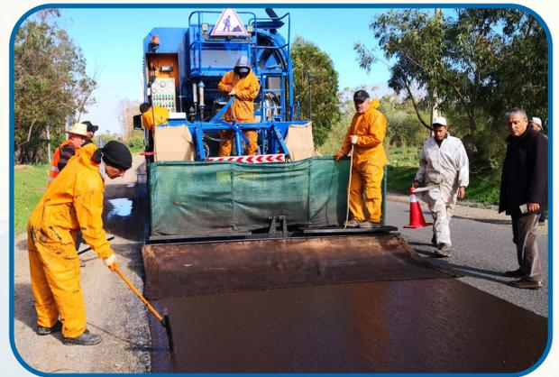
*Microsurfacing/slurry seal* is used commonly all over the world in many places from concourses to highways, airports, parking lots and other coated surfaces. Slurry seal has gradually increasing use in maintenance programs of governments, local or federal bodies – including the army – since being effective and economic.
